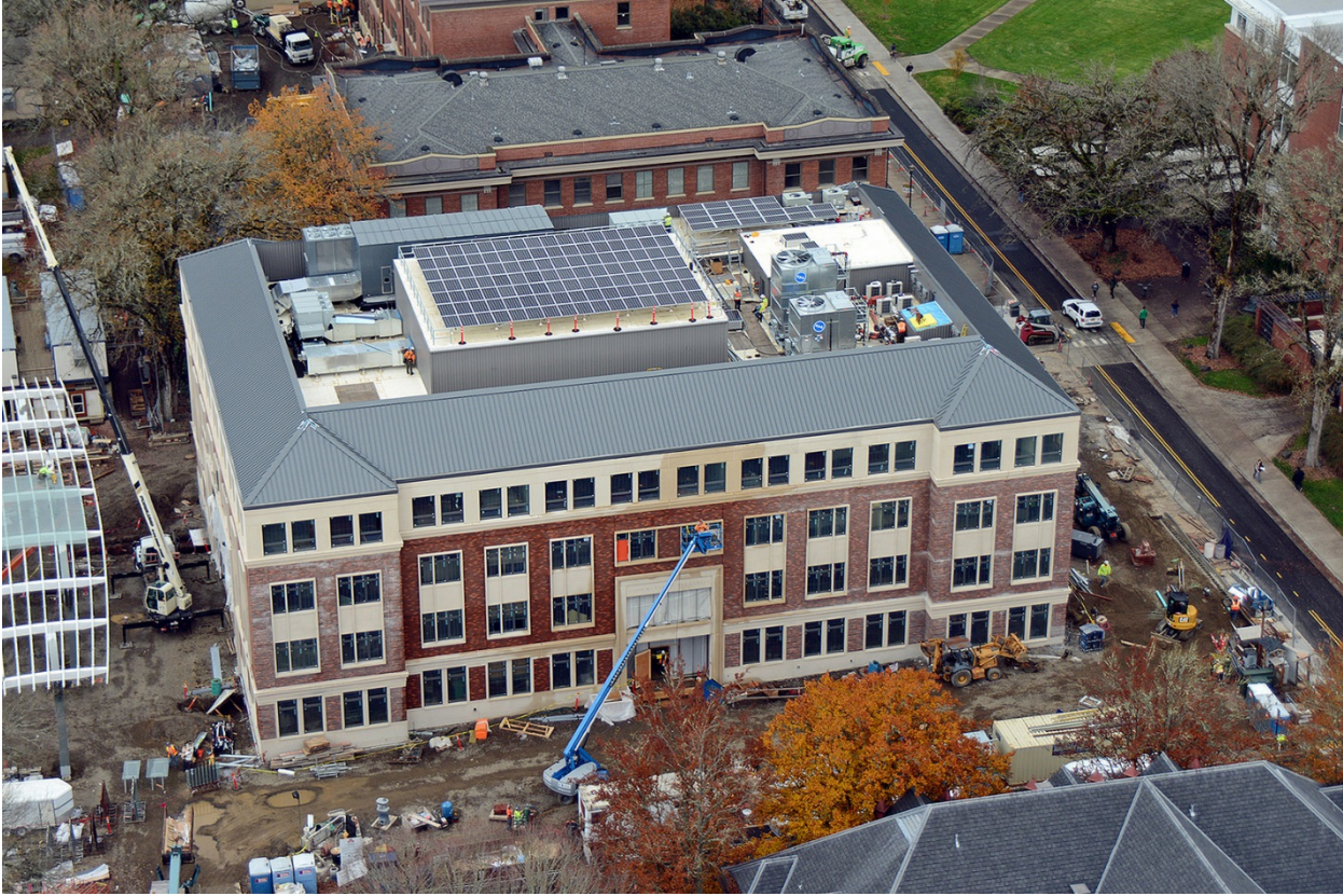
Student Experience Center under construction, including its 48 kilowatt solar array
